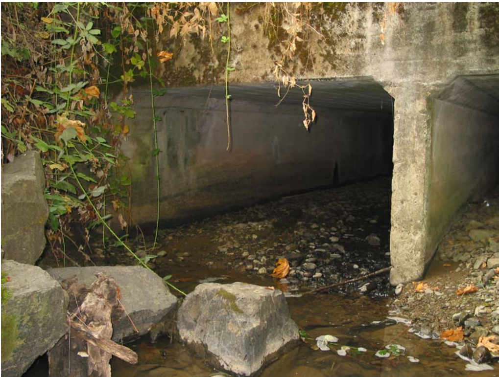
Figure 22. Culvert #1 outlet on Jordan Creek at I-5 (south half of twin box culverts).
