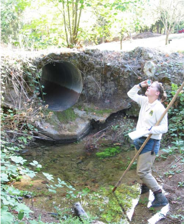
Figure 32. Culvert #9 outlet on Alder Creek at driveway off Meyer Lane.
