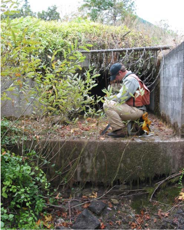
Figure 29. Culvert #7 outlet on Jordan Creek at Canyonville-Riddle Road.
