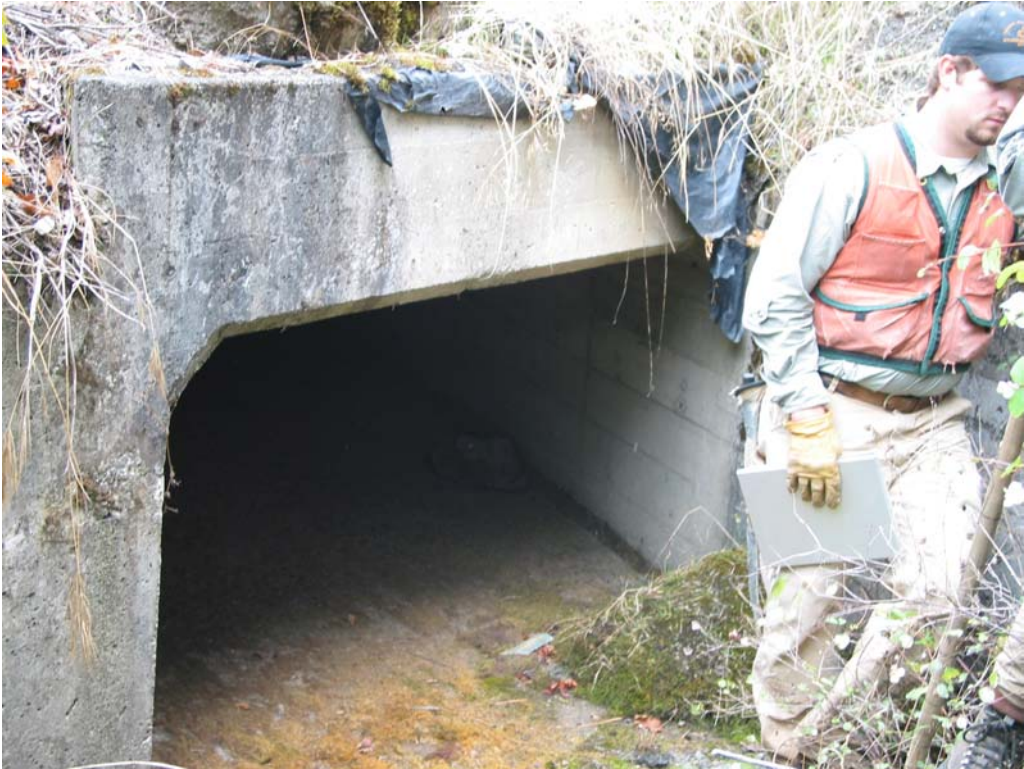
Figure 30. Culvert #7 outlet on Jordan Creek at Canyonville-Riddle Road.
