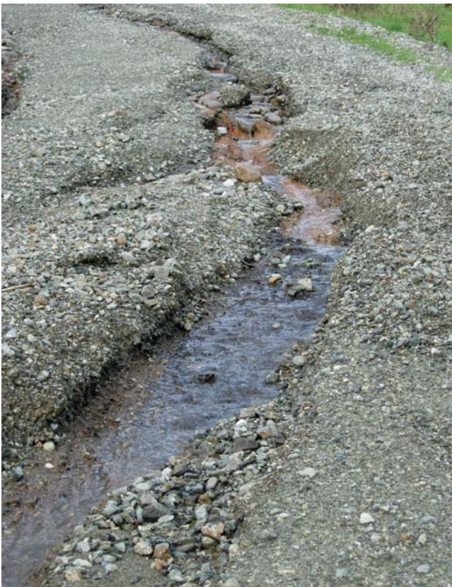
Figure 55. Erosion from driveway in Jordan/Alder Watershed.
